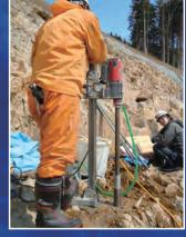
Drilling conditions using a simplified boring machine
