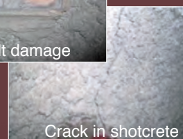
Damage to rock bolt (left) and crack in shotcrete (right) caused by action of strong earth pressure
